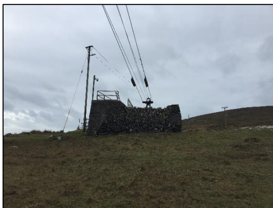
Plate 14.11: Island-side landing platform
