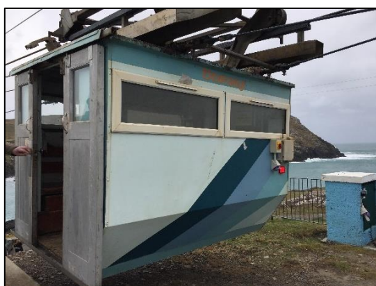
Plate 14.17: Cableway carrier cabin
