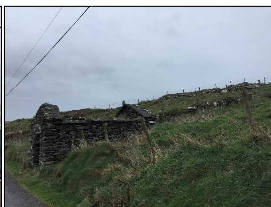
Plate 14.18: CH 36 ruined 19th century structure (mainland)
